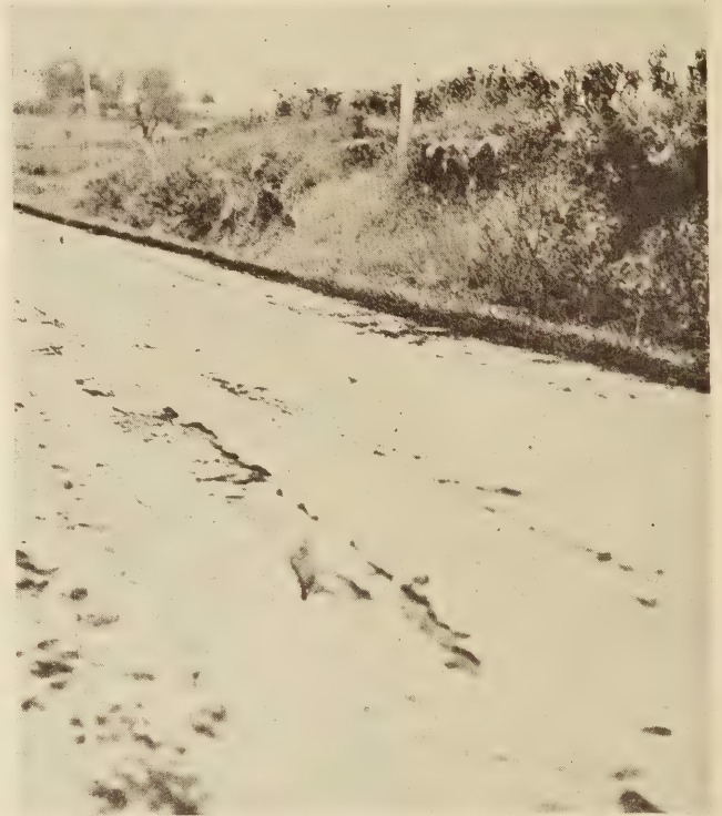
FIGURE 8.—MUTILATING EFFECT OF TRAFFIC AFTER RETREATMENT
